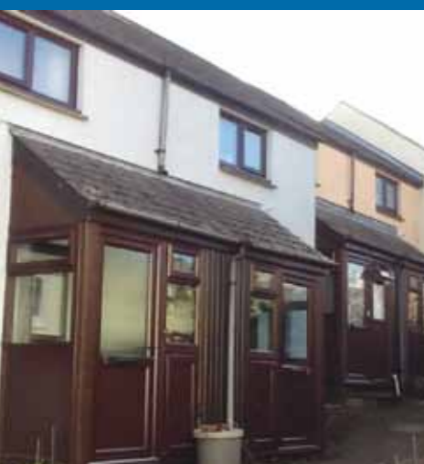
Properties at Grove Close Totnes had new windows and doors.
