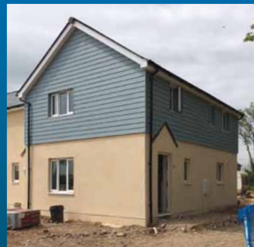
Four new family homes being built in Moreleigh.
