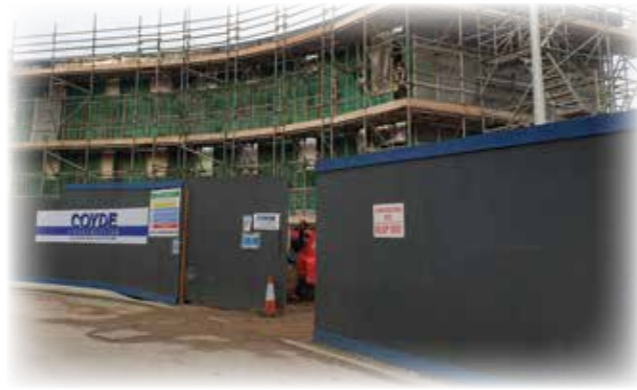
The 11 apartments are progressing well
