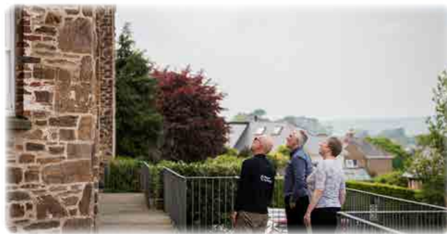
Inspecting Broomborough Court, Totnes.
